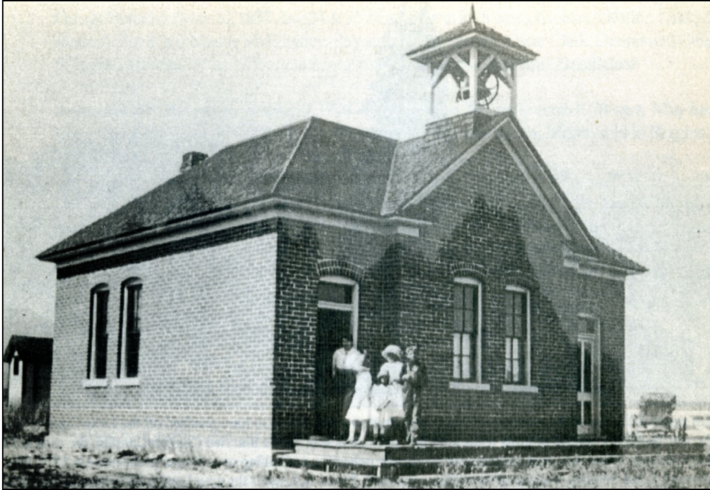
Figure 2. This ca. 1900-03 photograph of the Gas Creek School (view northwest) shows the original 1889-90 building and demonstrates that the same design was followed in the 1909 rebuilding. The image shows a full-width wood deck across the front and a privy at the left edge. Courtesy of Shaputis, Where the Bodies Are in Central Chaffee County, Colorado (1995), 37.
