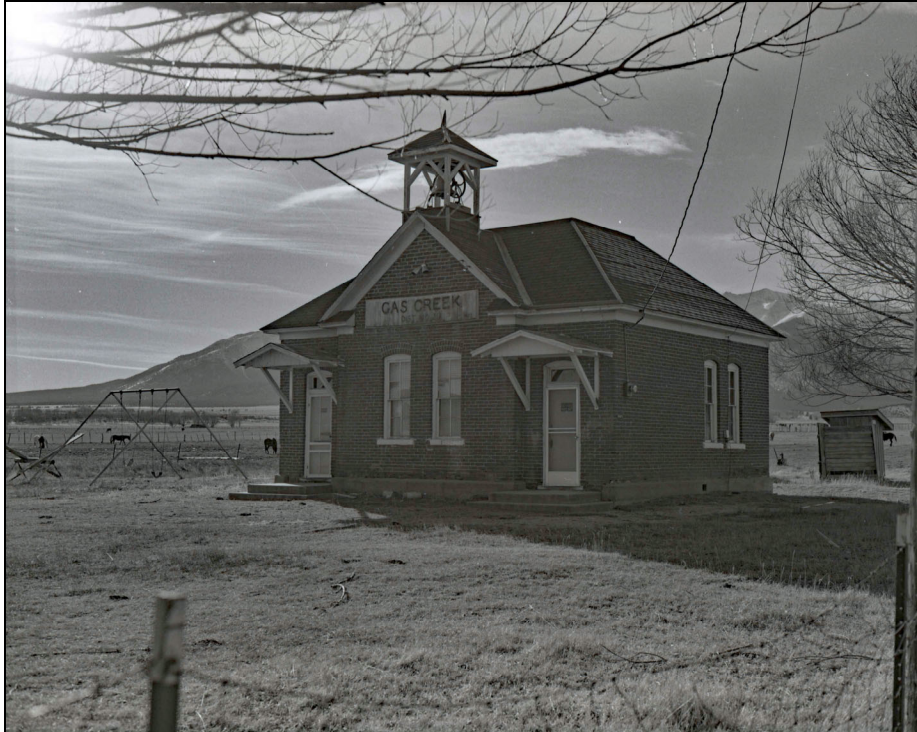
Figure 6. This view southwest in 1973 shows the school, privy (right), and playground equipment to the left. Courtesy of J. Todd, U.S. Bureau of Reclamation, 30 December 1973, Jean Hanfelt Collection, Salida Regional Library, Salida, Colorado.
