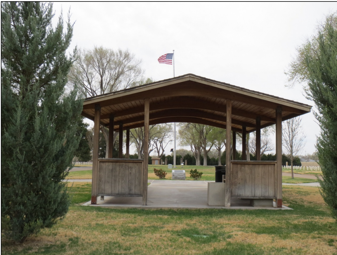
Figure 17. View looking south through the Committal Shelter to the cemetery entrance, 2004.
